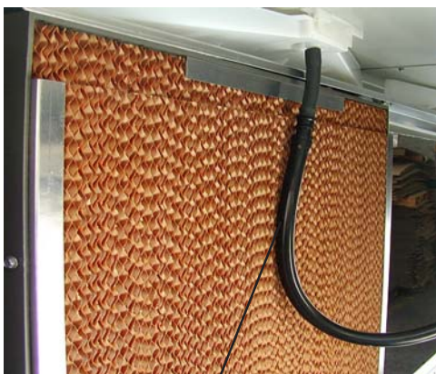
Incorrect length Water supply hose.
